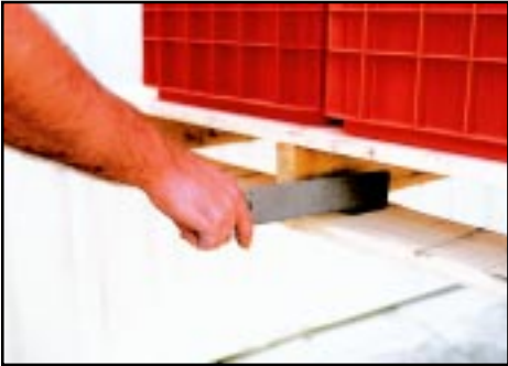
PLACE AROUND THE FIRST TWO-WAY STRINGER
